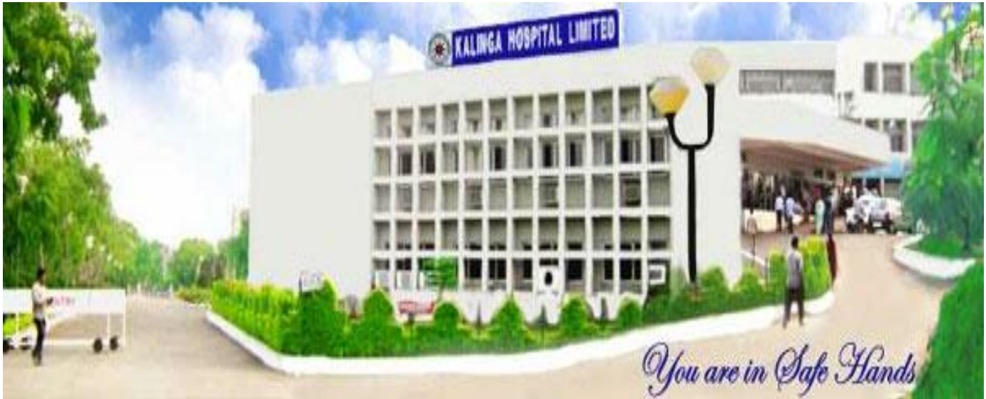
Lighting Illumination at Kalinga Hospital, Bhubaneswar, Odisha
