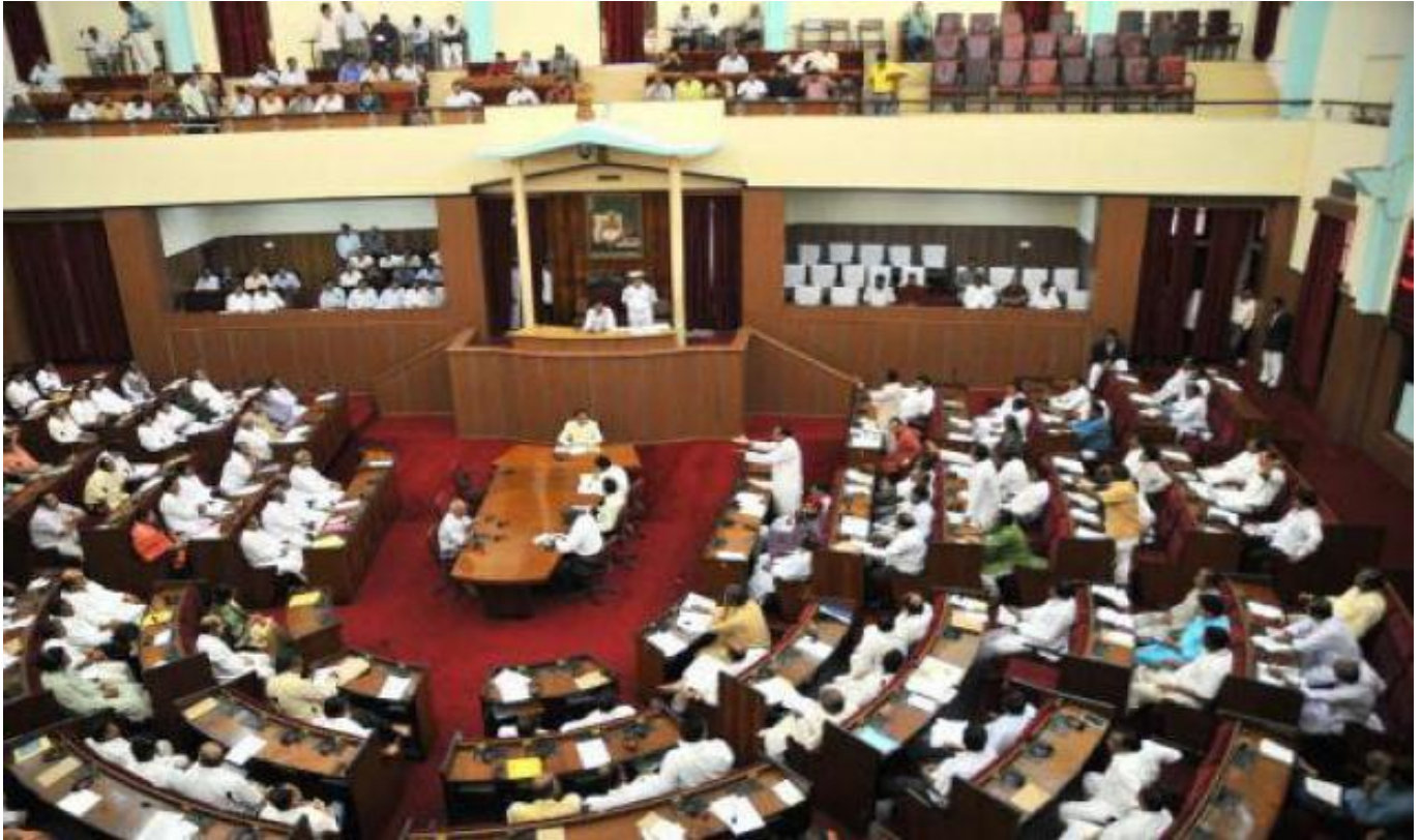
Lighting Illumination at Odisha Legislative Assembly Hall (OLA), Bhubaneswar,
