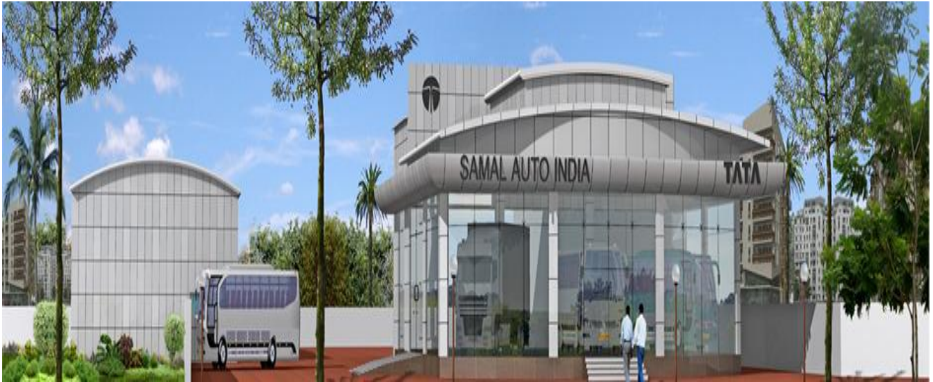
Lighting Illumination at Samal Auto India, Banarpal, Odisha
