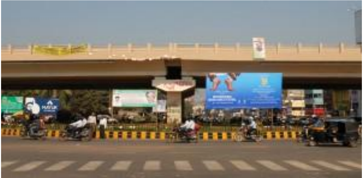
Lighting Illumination at Rajmahal Square, Bhubaneswar, Odisha
