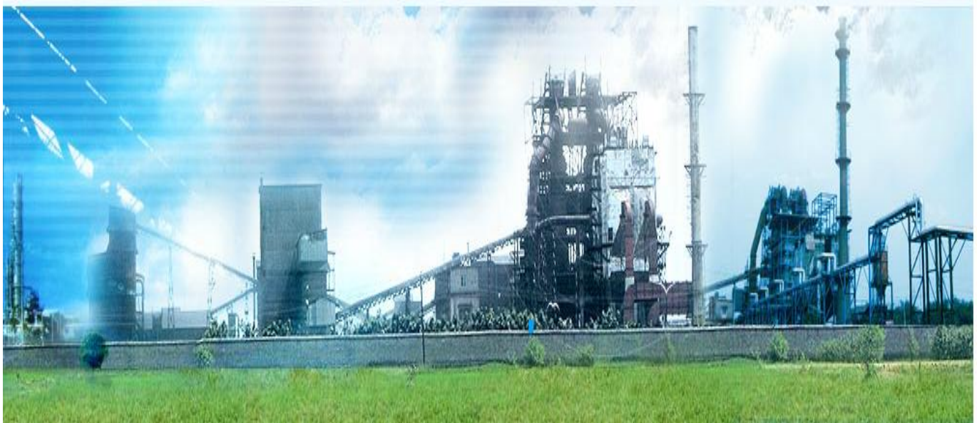
Lighting Illumination at Scan Steels Ltd, Ramabahal, Odisha
