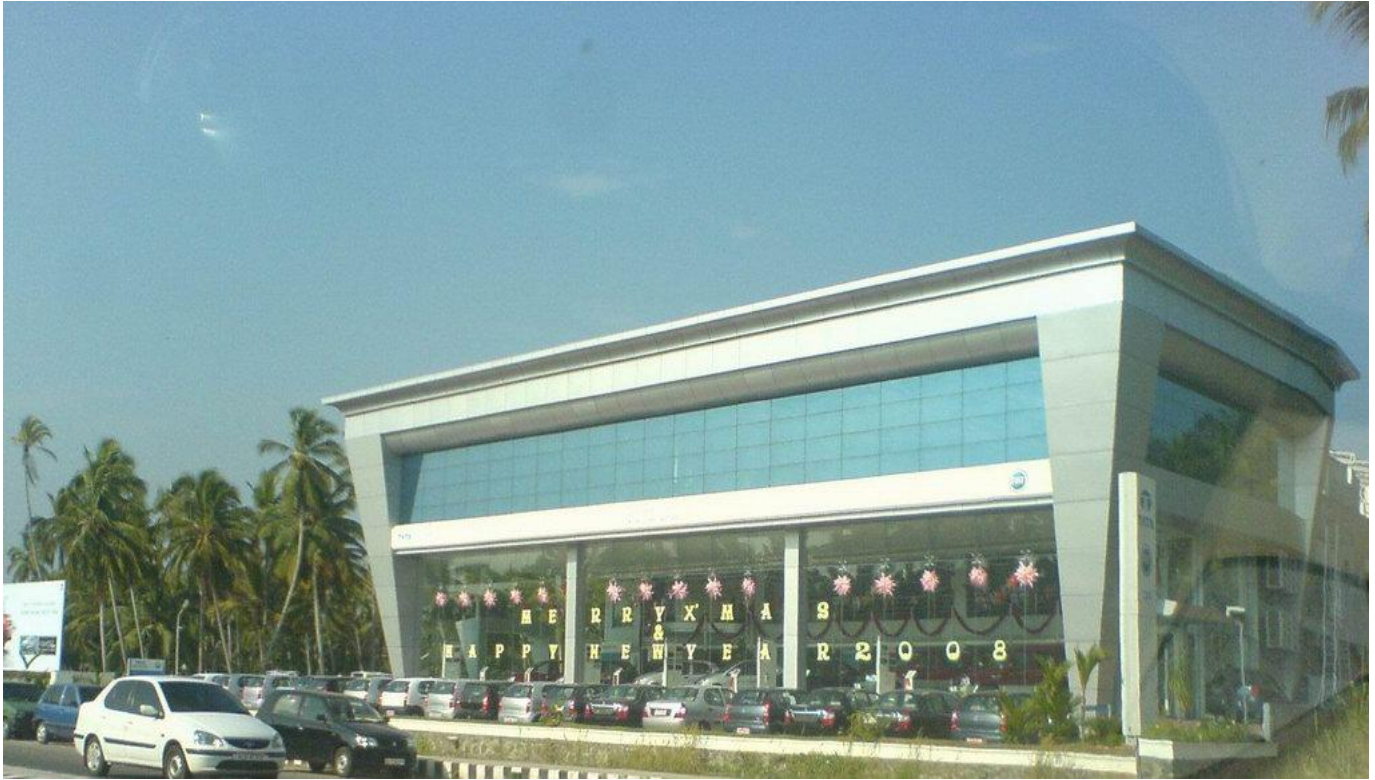
Lighting Illumination at Trupti Automotives, Cuttack, Odisha
